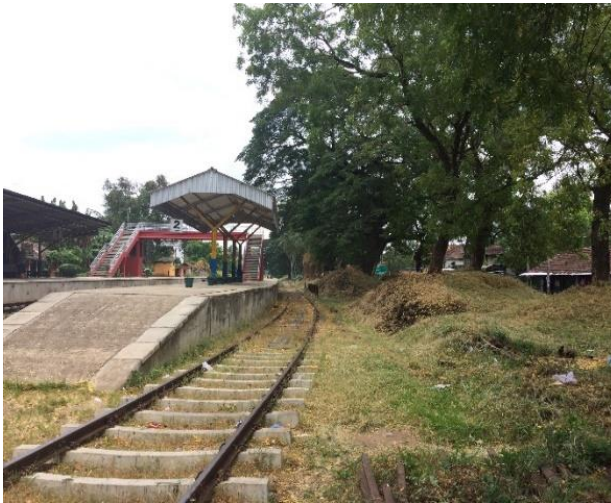
Existing condition of Wellawa railway station
